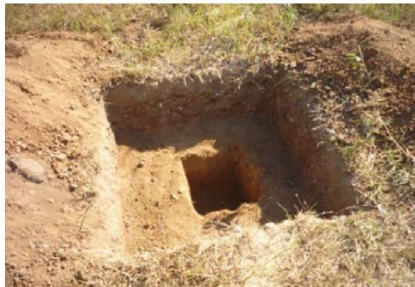
Preparing a pit trench
